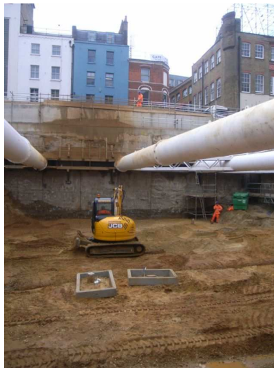
General view of bulk dig, looking west
