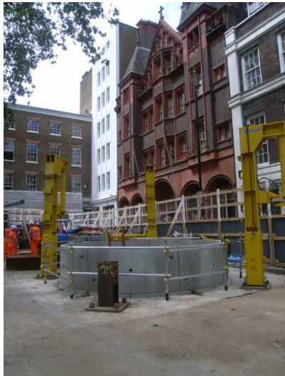
Grout Shaft 2, general view, looking NW
