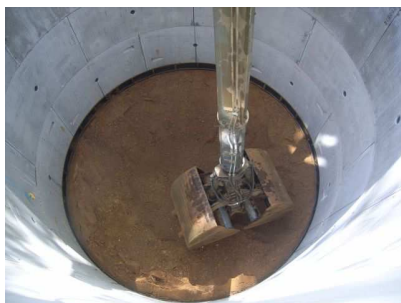
Grout Shaft 2, natural deposits, mid depth
