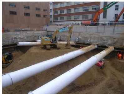
General view of bulk dig, looking SW
