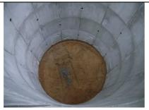
Grout Shaft 3, lower gravels and London clay
